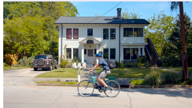
Historic Single Family Conversion, Decatur, Georgia
