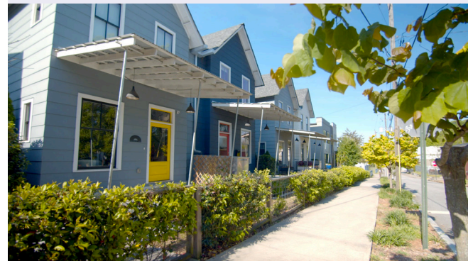
New construction duplexes, Reynoldstown, Atlanta
